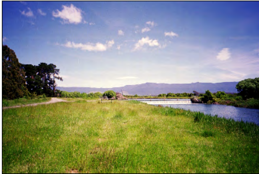
Photo 4.3 Weir 2, car park and picnic table, looking upstream from Lees Bridge.
