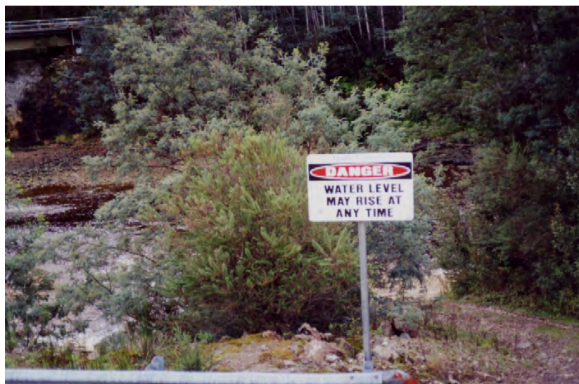
Photo 5.16 Public Warning Sign on the King River immediately downstream of John Butters Power Station
