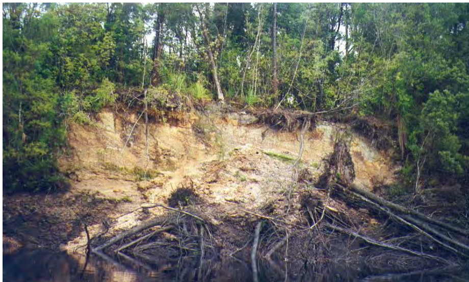
Photo 3.7 Ground level view of recent landslip between Abel Gorge and the Splits under low water conditions
