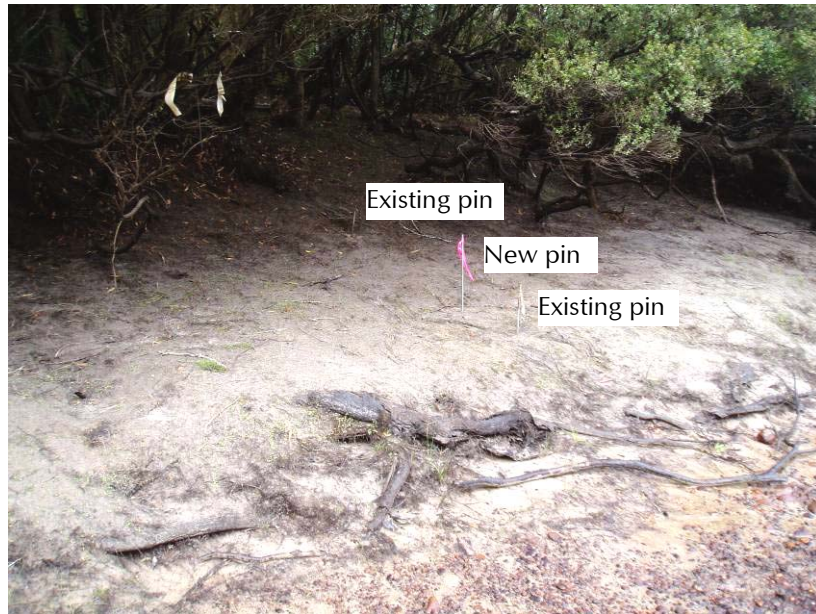
Photo 1-1. Erosion pin site 21 showing placement of new erosion pin on bank
