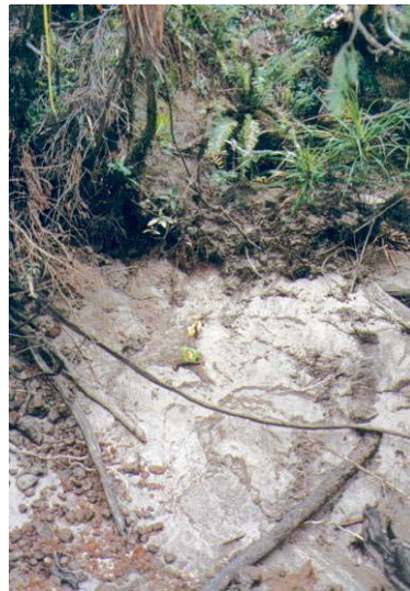
Pin 3B/1 and scour chain December 2001
