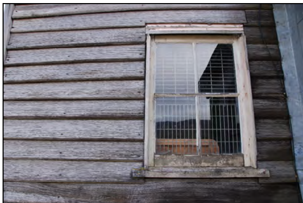
Photo 56: Window 1, eastern elevation.
