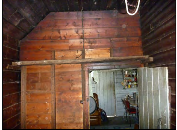
Photo 38: south west room looking north with slab bench above door.
