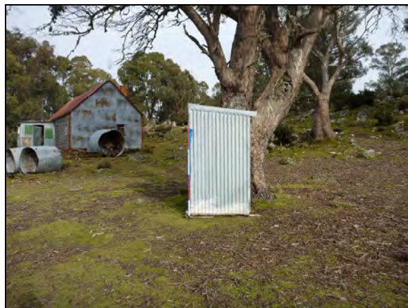
Photo 50: outhouse, eastern elevation.
