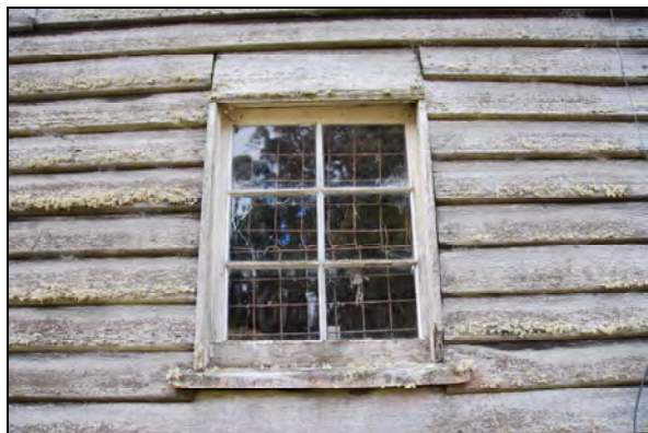
Photo 55: Window southern elevation
