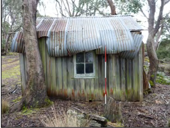
Photo 2: Southern elevation of hay shed, with single window and any overhanging sheets of corrugated iron.
