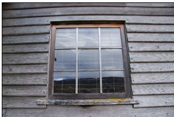
Photo 57: Window 2, eastern elevation.
