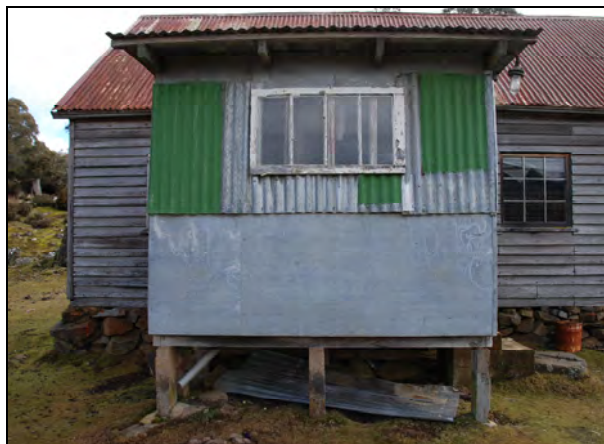
Photo 18: Porch, from east.
