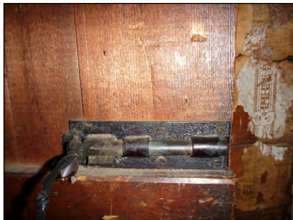
Photo 28: south east room lock, inward side of door.
