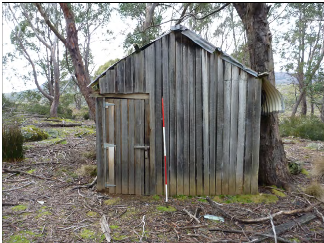
Photo 1: Western elevation of the hay shed with entrance door.
