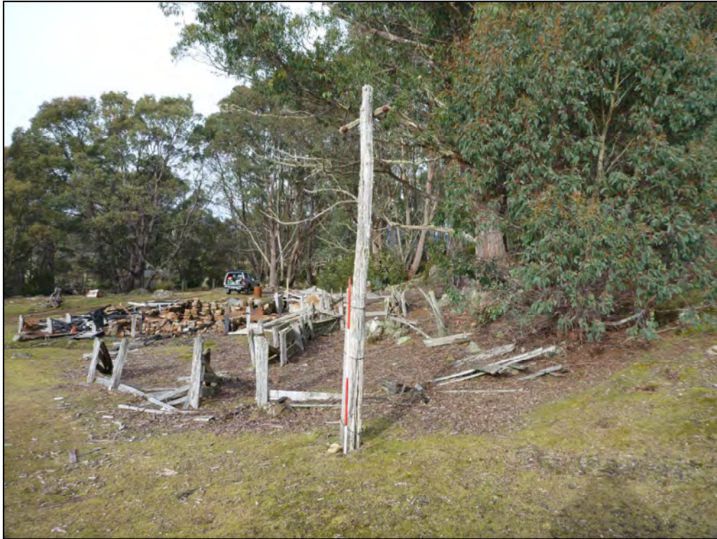
Photo 45: Power pole, looking south.
