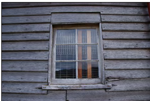
Photo 58: Window 3, eastern elevation.
