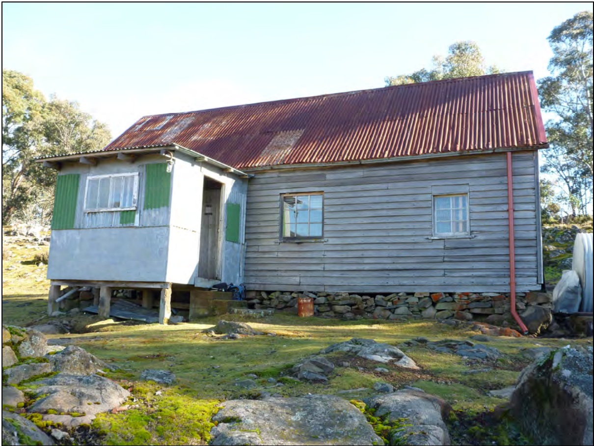
Photo 11: Eastern facade of Bye's House.
