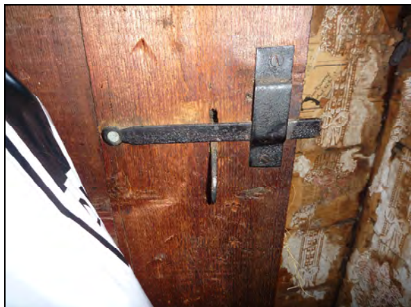
Photo 27: south east room latch, inward side of door.
