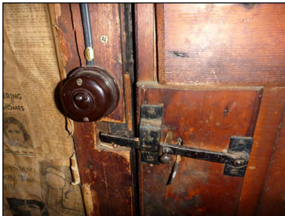
Photo 25: north east room latch, inward side of door.
