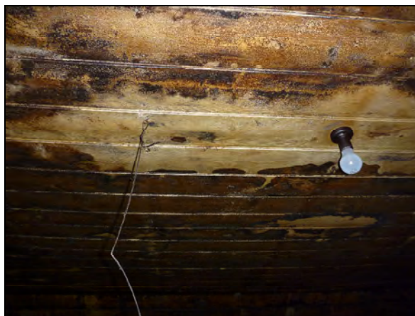
Photo 29: wire from ceiling, reportedly for preparing snares.
