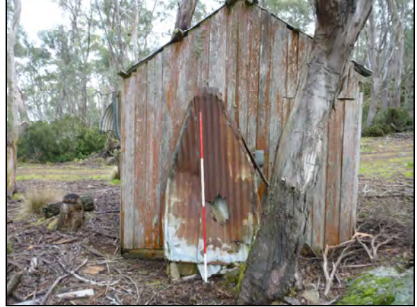
Photo 3: Eastern elevation of hay shed, with chimney base, and blocked off second entrance.
