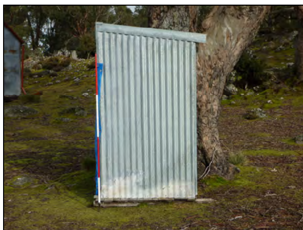
Photo 51: outhouse, eastern elevation.
