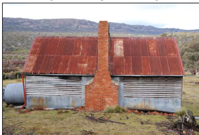
Photo 16: western wall with combination materials.
