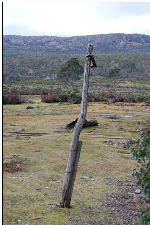
Photo 46: Power pole, looking east.
