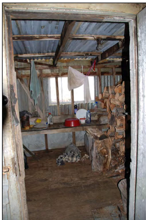
Photo 23: interior of porch, looking from central living space.
