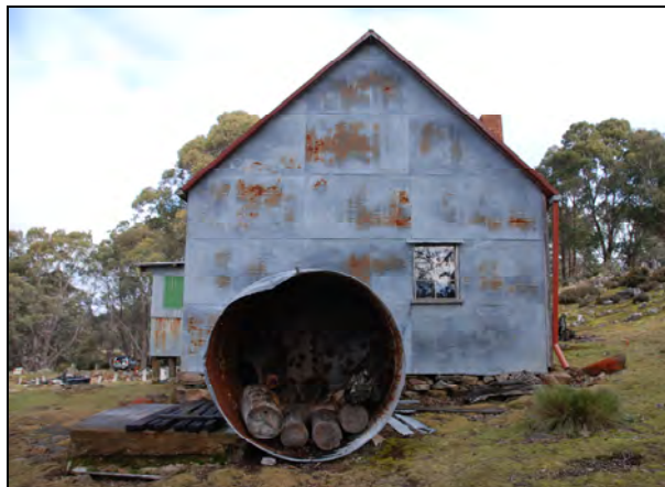
Photo 47: water tank and stand.
