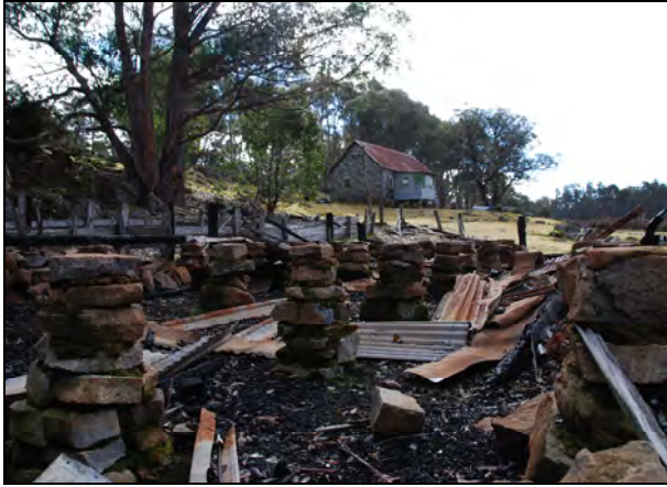
Photo 6: Stone piers of the shearing shed.
