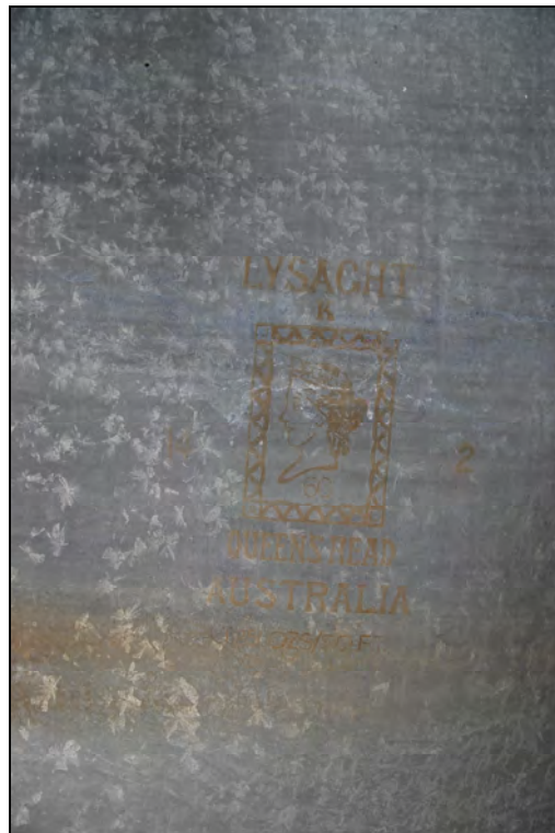
Photo 13: Detail of Lysaght sheeting.
