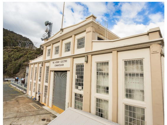
Figure 25: Tarraleah Power Station
